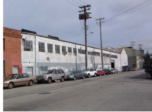
View toward northeast, 11.16.07, 100_1865.JPG
